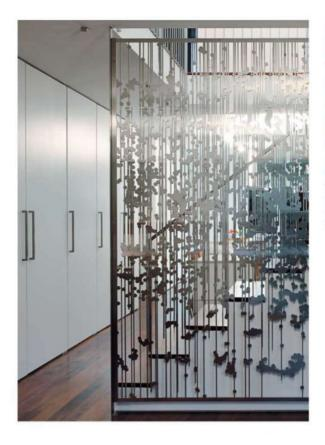
Andrew Magnes's hanging screen (this page), composed of aluminum circles and lines, cut with a CNC water jet, separates the entry from the staircase and rear kitchen area. To accommodate his passion for cooking, Renaldi (opposite bottom) insisted on the long Carrara marble countertop, a niche for cookware (opposite top left), and ultracontemporary appliances.
